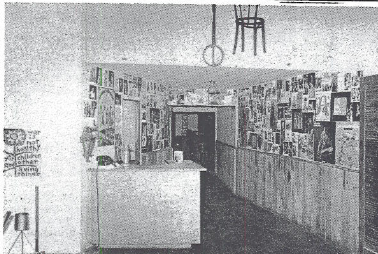
In sharp contrast to the charred walls in last week's photo, the Ash Grove is now very much back in business after a quick overhaul by painters, carpenters and electricians.
