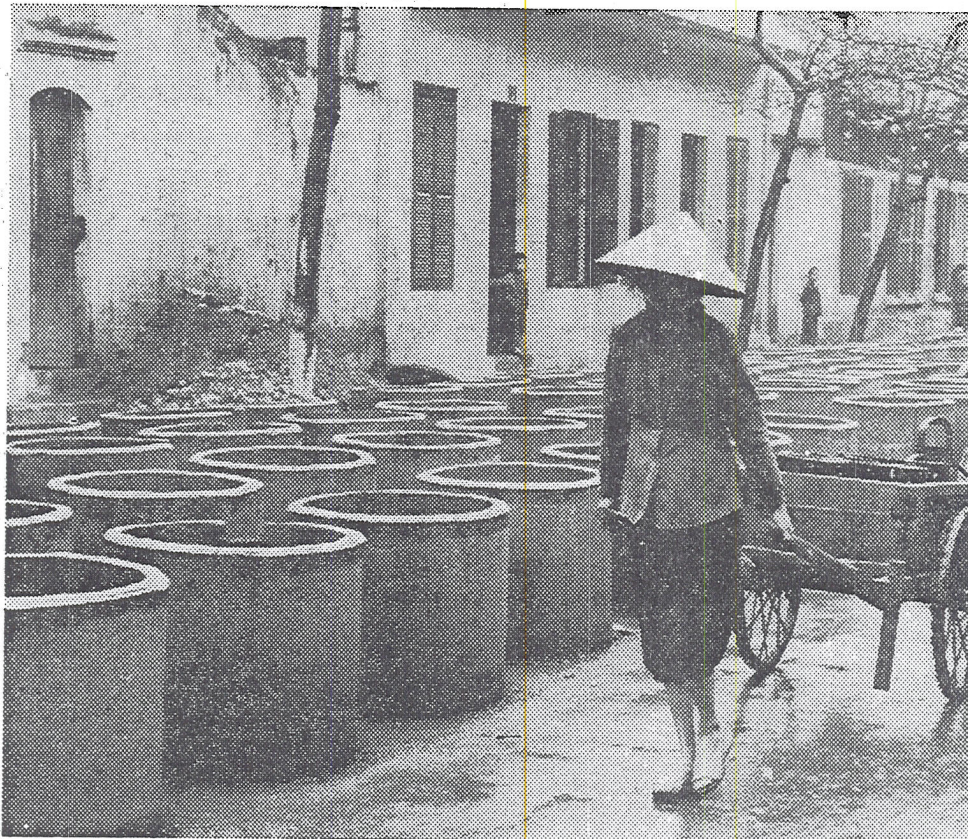
READY FOR DEPLOYMENT: Concrete tubes used in air-raid shelters lined up in Hanoi, North Vietnam's capital have them and workers are digging holes for sinking new ones as bom-
