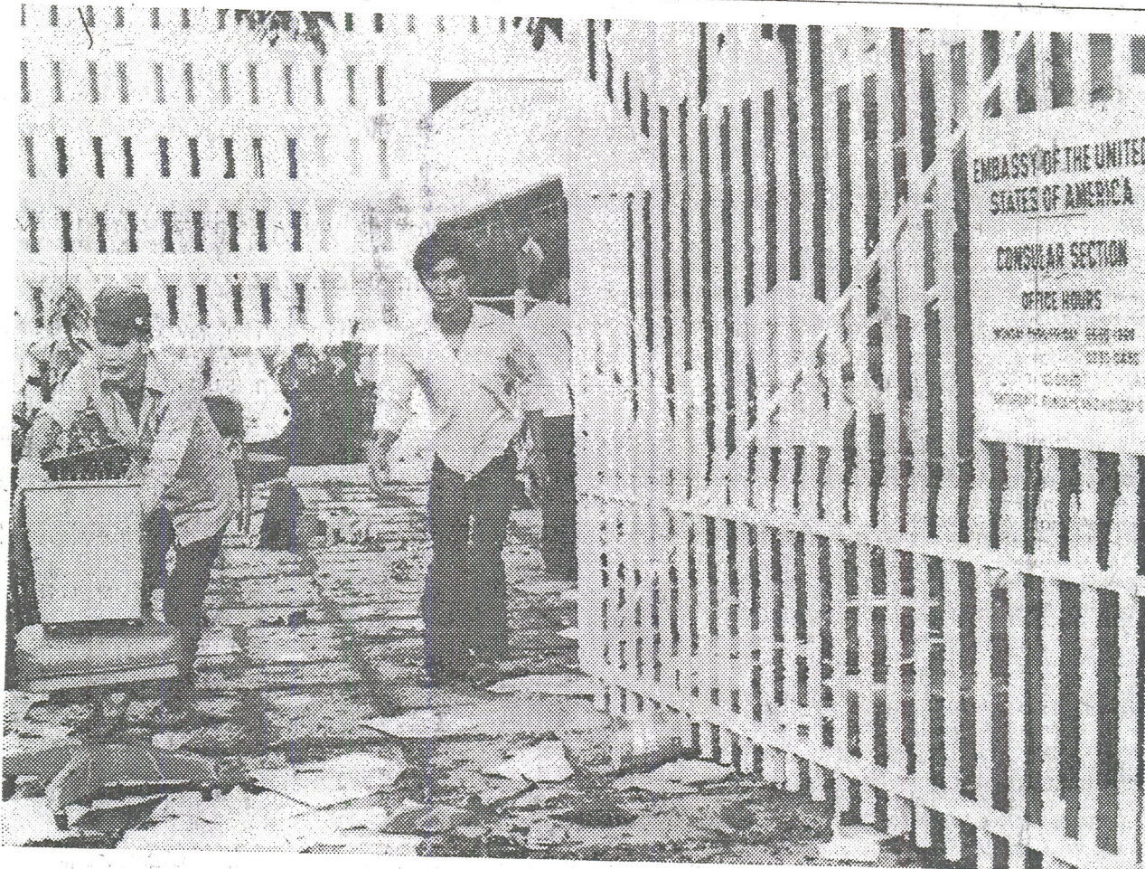
South Vietnamese were quick to remove furniture, plumbing fixtures and other property from the U.S. Embassy in Saigon on Tuesday after it was evacuated and the security guards left the premises. United Press International
