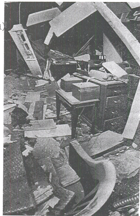
DAMAGE AT STATE DEPARTMENT BUILDING A tired and counterproductive tactic.
