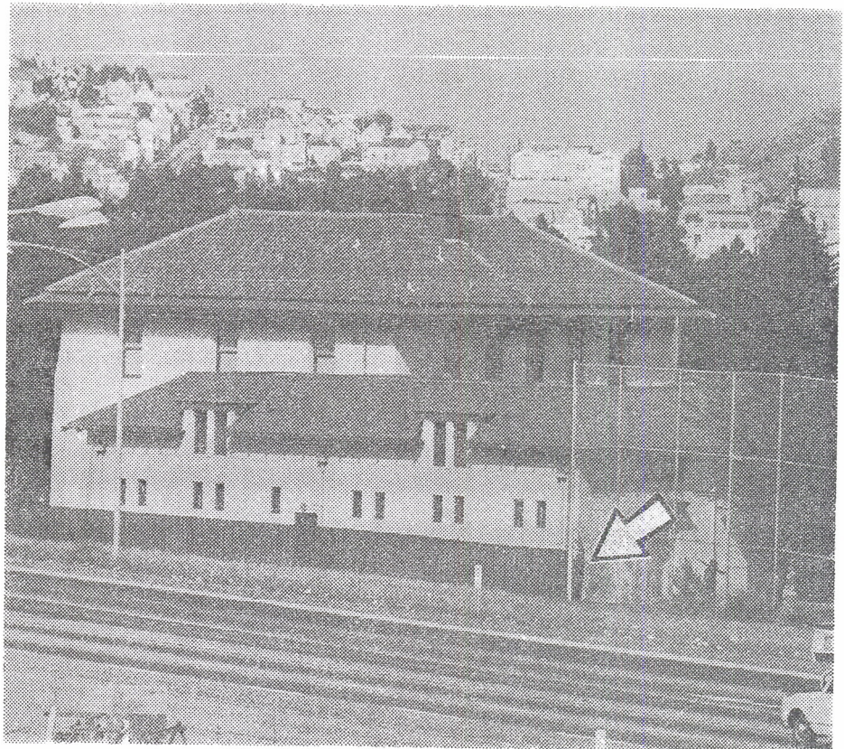
A shotgun-armed guard patrolled near the spot (arrow) where a hole was cut in the Ingleside station's protective fencing
