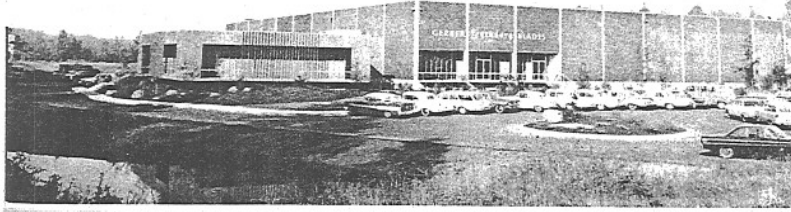
Gerber Legendary Blades, main office and manufacturing plant, Portland, Oregon
