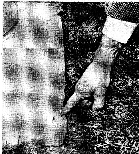
BULLET MARK in the concrete is pointed out by author, who claims angle of groove made by bullet proves it couldn't have been fired from book depository.
