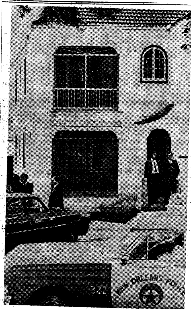
DAVID FERRIE'S APARTMENT at 3330 Louisiana ave. pkwy., where the flying instructor-private investigator was found dead yesterday.
