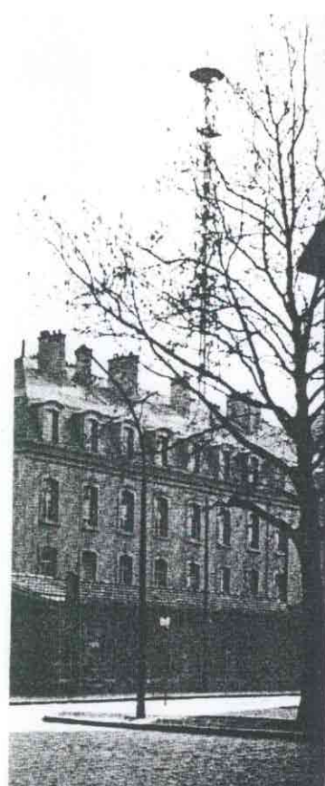
SDECE headquarters in Paris, a former army barracks, is topped by a huge communications tower.
