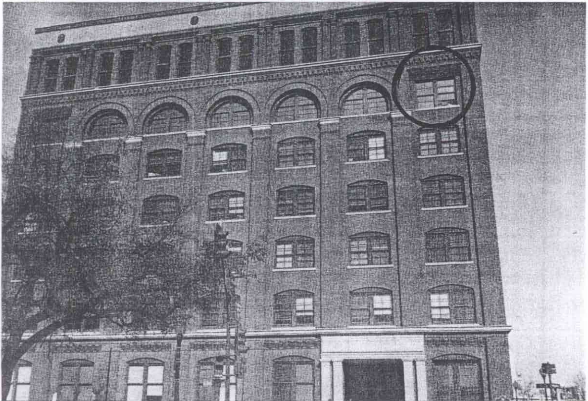
NOTE: SIXTH FLOOR WINDOW CIRCLED PHOTO: HARRY YARDUM
