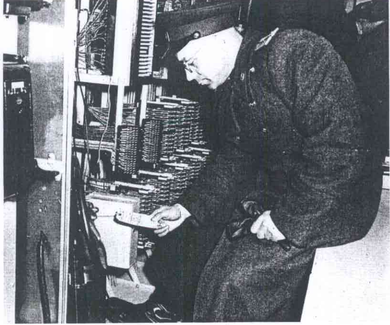
Super spy's activities nearly drove Reds crazy. Here, Russian officer inspects elaborate tapping switchboard found in tunnel to East Berlin.
